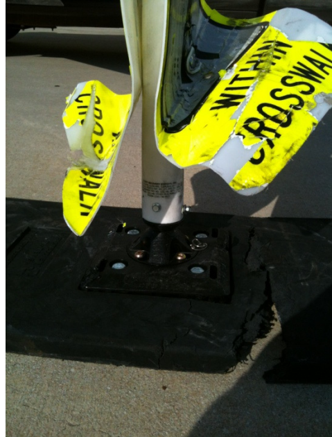
Figure 3 - Tested to Failure Mode
